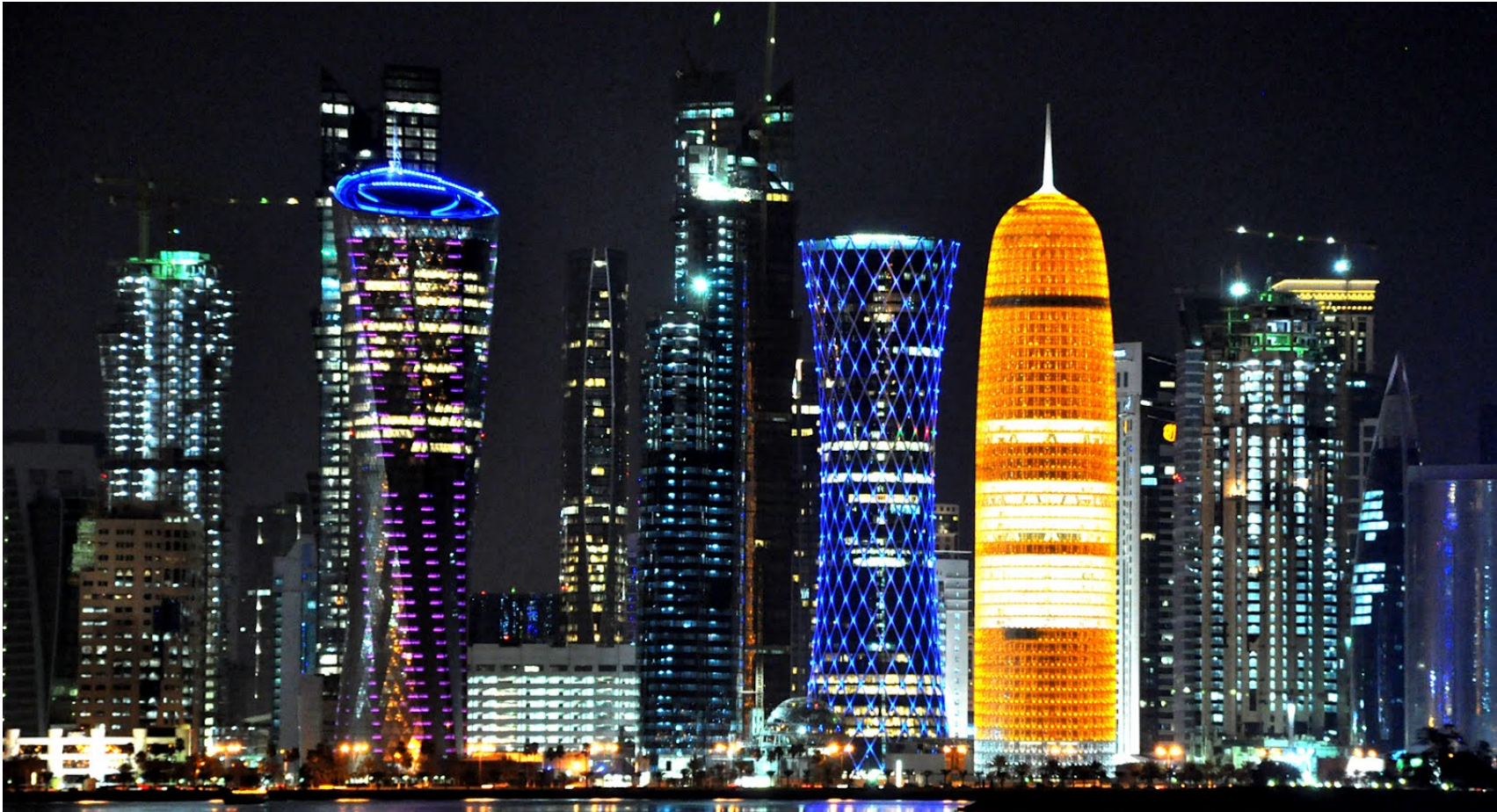
Low-energy light-bulbs in Doha
